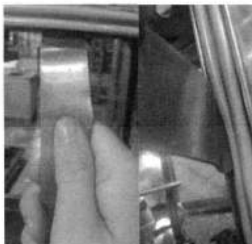
Figure 41 – Gasket removal
