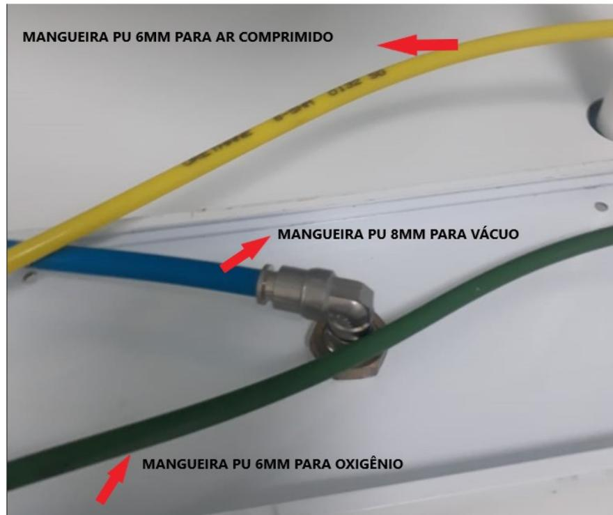
*Figura 12 – ITEM 14/15/17: MANGUEIRA PU 6MM COR VERDE PARA OXIGÊNIO / MANGUEIRA PU 6MM COR AMARELA PARA AR COMPRIMIDO/ MANGUEIRA PU 8MM COR VERDE PARA VÁCUO*
